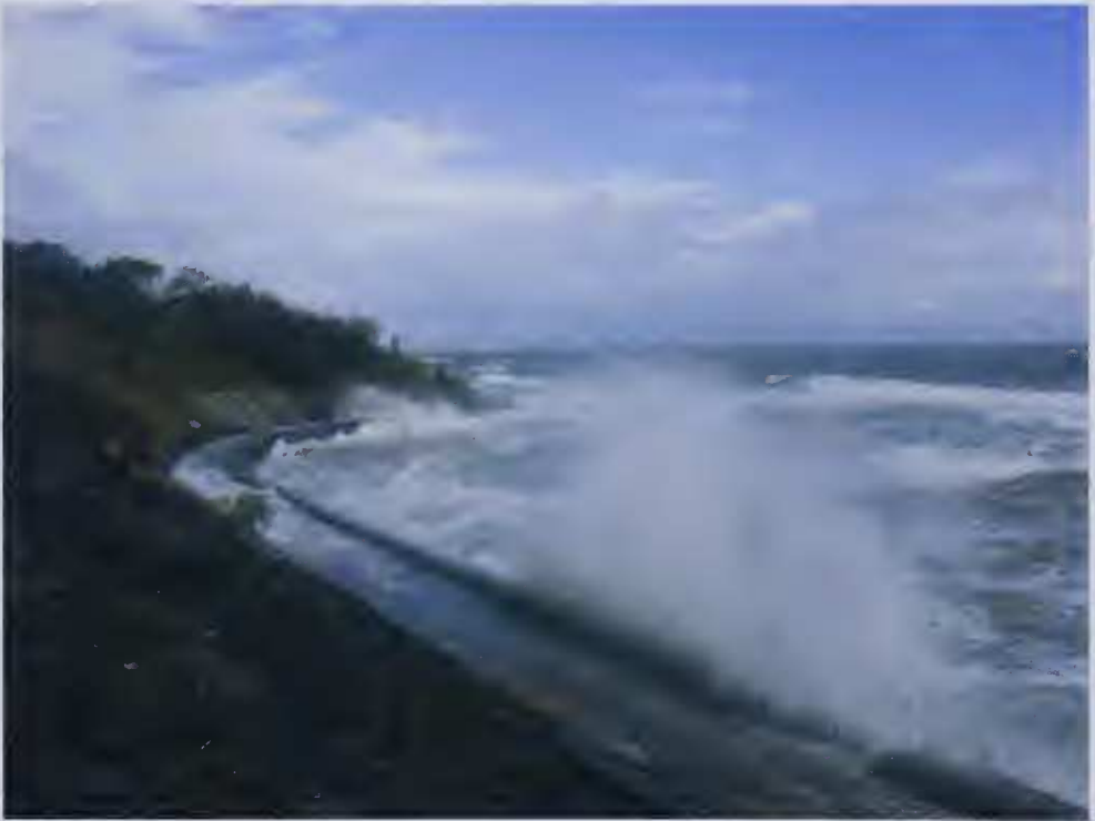
Fig. 3. Waves breaking over the sea wall at Quiet Corner on 26 April 2009.
